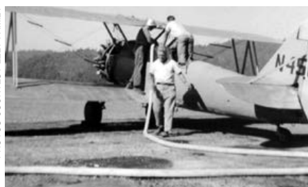
ABOVE: Wim Lely, Martha's dad, pumps retardant into a Stearman biplane in the late '50s. He developed Fire-Trol, the early retardant mixture, as well as the locking valves that attach the pressurized hose to the plane. LEFT: Gary and Martha Soeth on their wedding day, 1965. Dad would call within days to pull them from their honeymoon to load retardant for a fire in Beckwourth, Calif.
